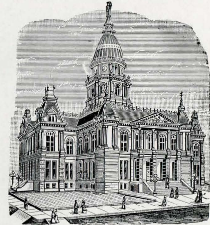
Tippecanoe County Court House
